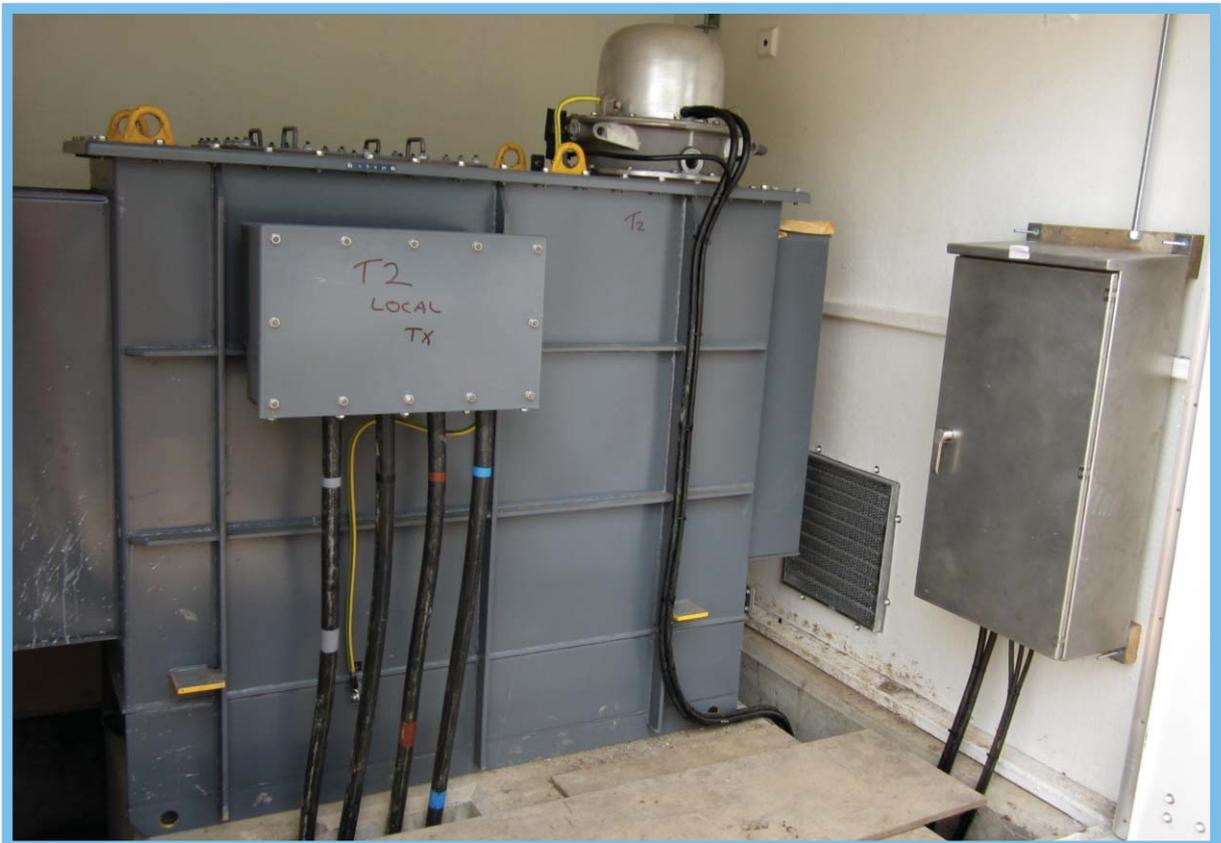
Distribution transformer with on-load tap changer: one of the first UK installations
